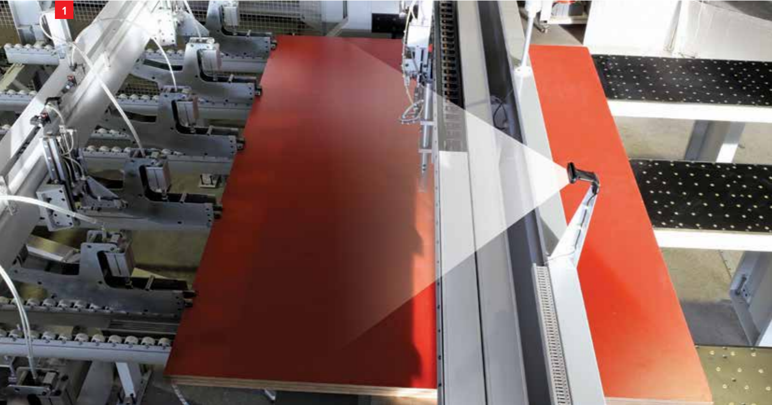
1 Kamera Sistemi Loading Zone Monitoring
